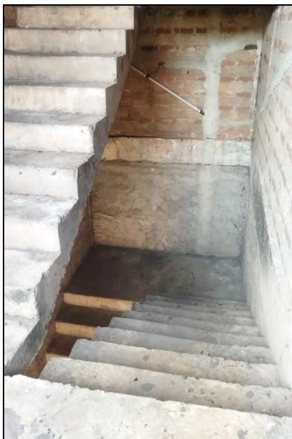
Figure 3 - The Staircase of one of the flats
